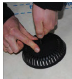
Overdelen presses ned mod undertaget.
